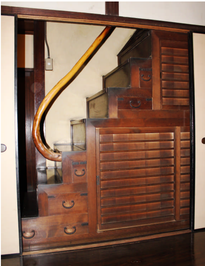
Fig. 18 Handrail probably added at a later stage Kojima house, Kyoto (photo Karel Bos)
