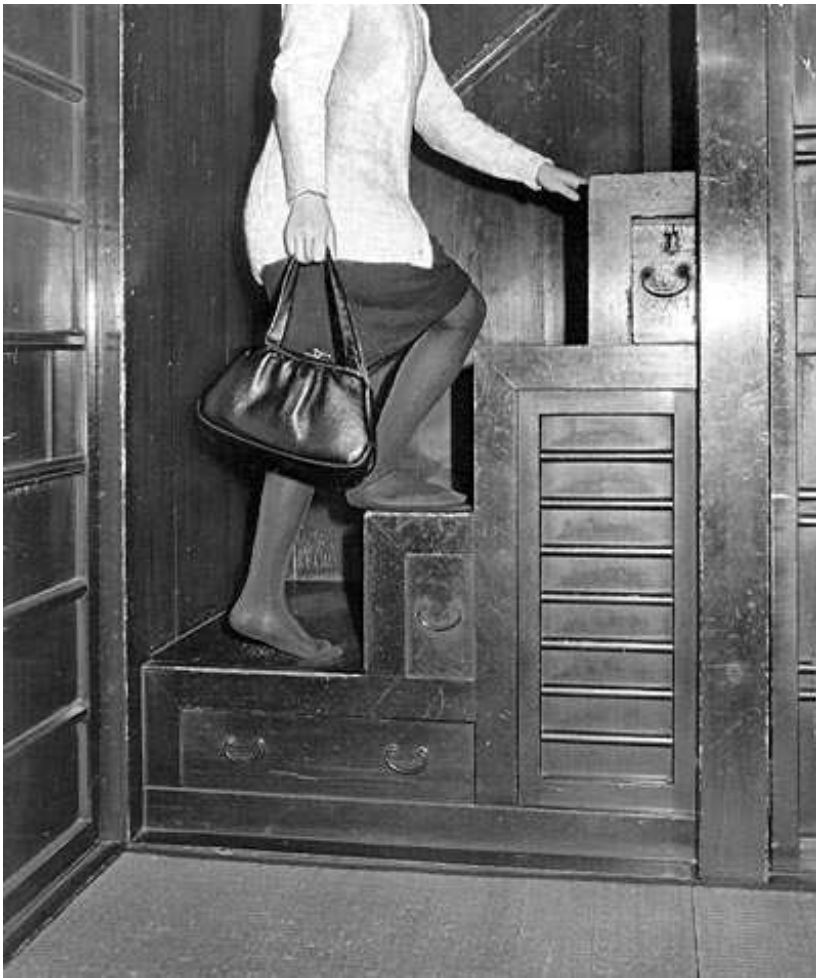
Fig. 30 Access from the side via a widened step
