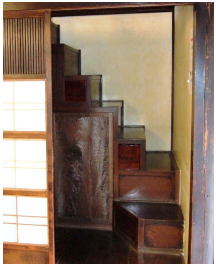
Fig. 12 + 13 Arrangement of the steps when approach from the front of the chest is required (photos http://www.kyotomachiya.com )
