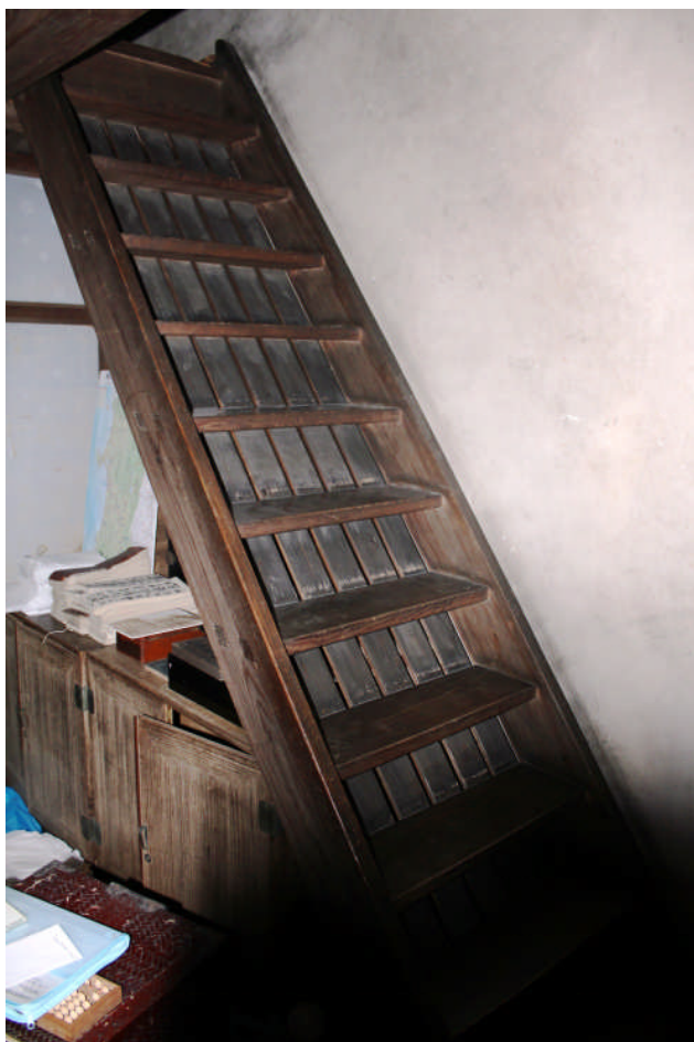
Fig. 8 Stair-ladder (photo Karel Bos 01/11)
